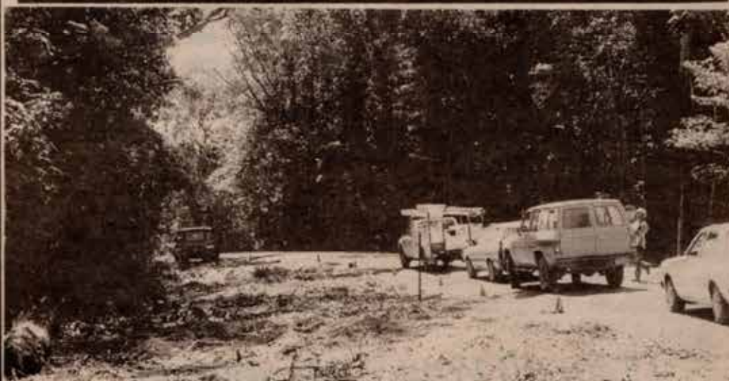
Myola roadworks and water main construction.
