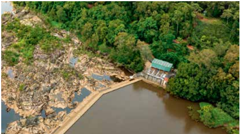
Above: Kuranda Weir pictured before Ex-Tropical Cyclone Jasper. Below: Flooding events associated with Tropical Cyclone Jasper caused the Kuranda Weir embankment to be washed away, rendering the Barron Gorge Power Station inoperable for six months.
