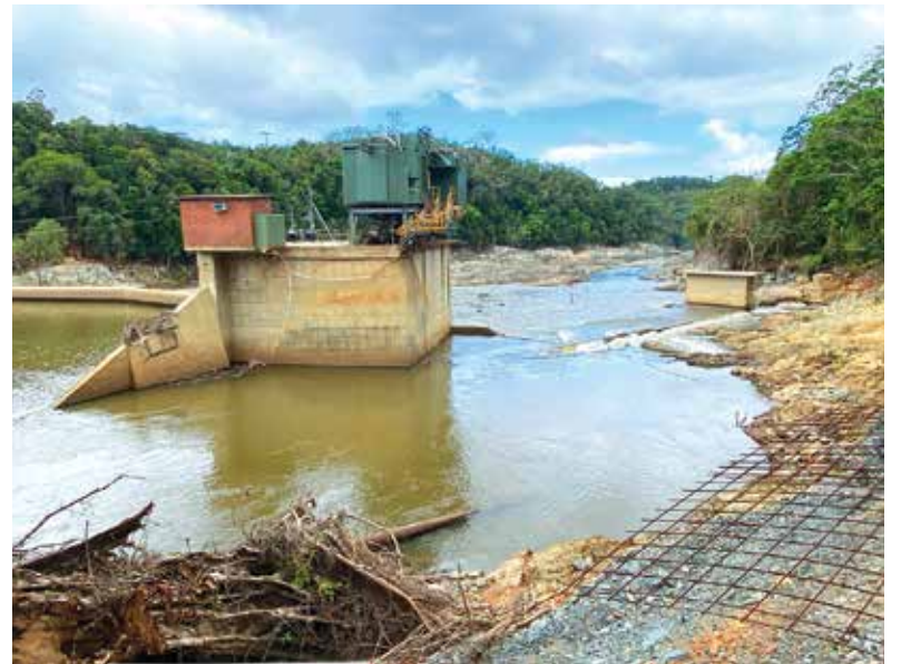
Tackling damage at the Kuranda Weir following flooding in the wake of ex- Tropical Cyclone Jasper in December 2023. Photo CleanCo. The Kuranda Paper December 2024.
