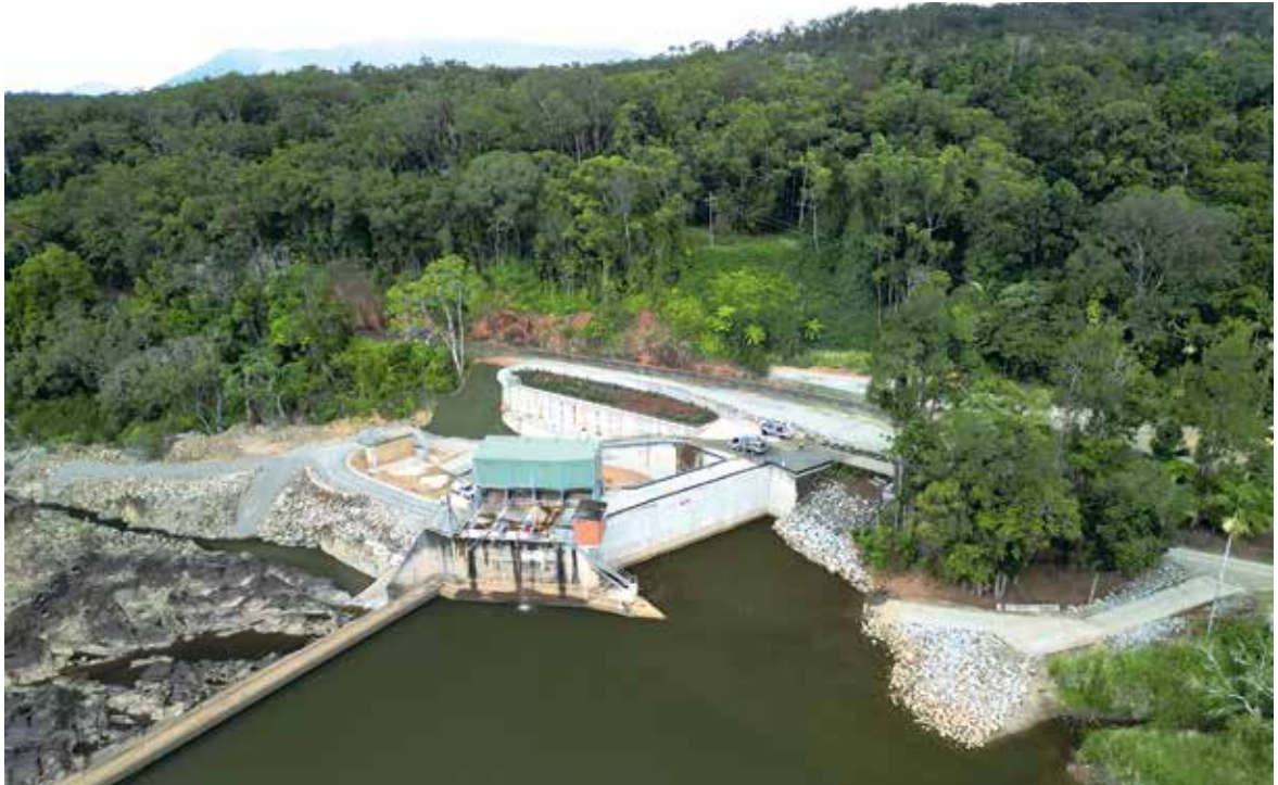
The Kuranda Weir Recovery Project was officially completed in September 2026. Photo Credit: Chris Leach.
