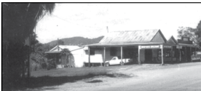
Foodland Store before restoration CHS PHOTO
