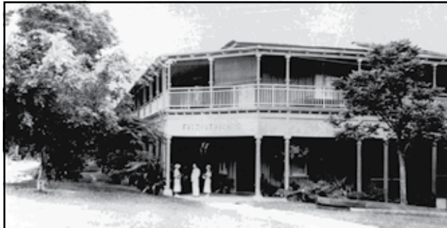
Fitzpatricks Tavern before restoration CHS PHOTO
