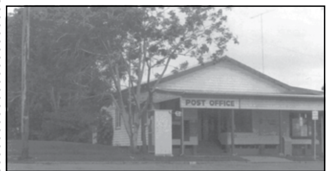
Kuranda Post Office CHS PHOTO
