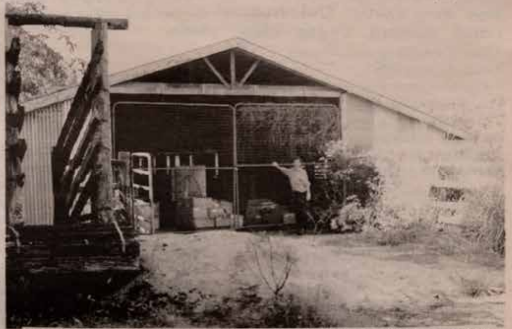
The Myola Road Stables where the new community Pottery Studio is being built.
