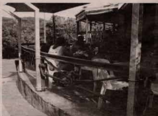
Balustrade made from railway iron over 120 years old, being used as a support for a bare metal and canvas canopy!
