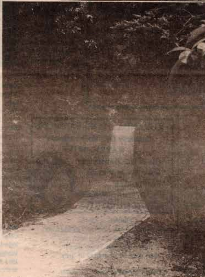
This is what has been happening in Rob Veivers Drive behind all that tall grass! We have been seeing rows of parked cars, large machines going in and out, and men with Stop and Go signs, all through the wet. New paving on the walking track is the result.
