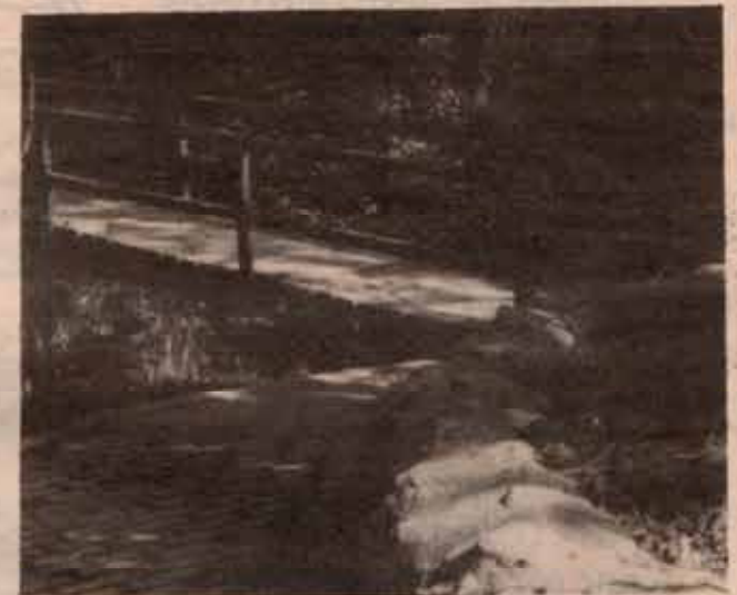
Newly completed bridge and path at Jum Rum.
