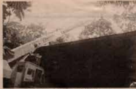
Removing Tree Off Roof
