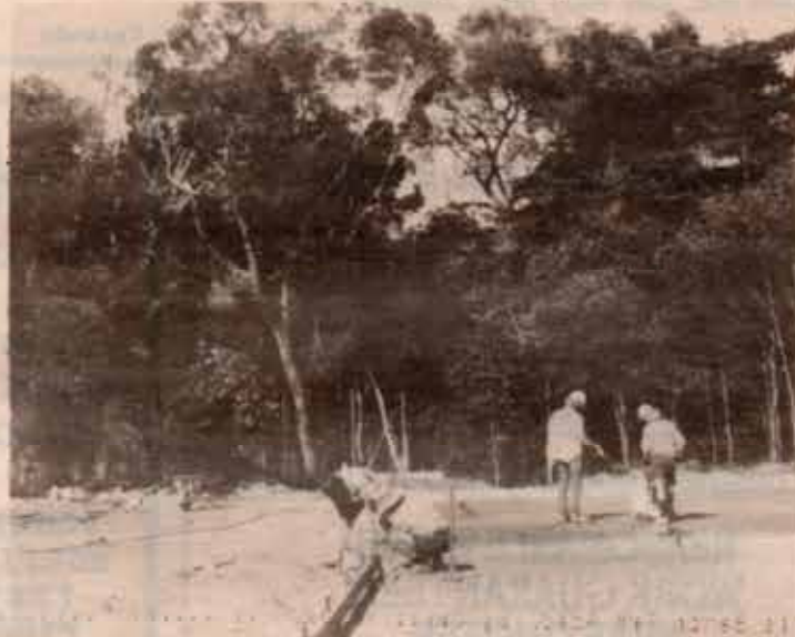
Basketball court near Kindy nears completion.
